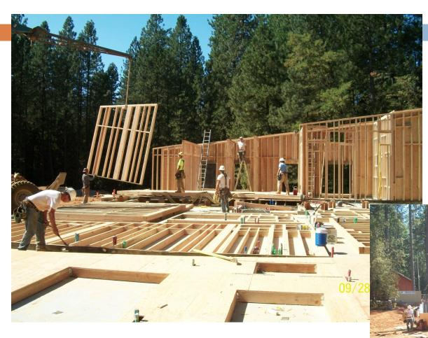
Individual walls were built on the ground and craned into position.
